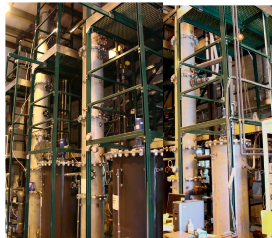
250 kW Chilled Ammonia Process Mini-pilot System
